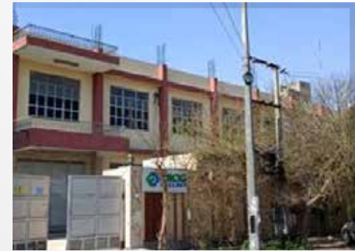
Noida: Service Office & Storage Facility
